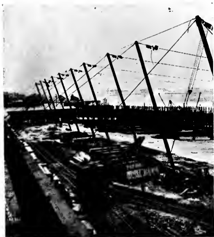
View looking south, showing trolley masts and locomotive crane in the foreground.
